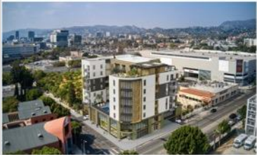
Link Apartments SM 1353 Western Los Angeles, CA 65 units
