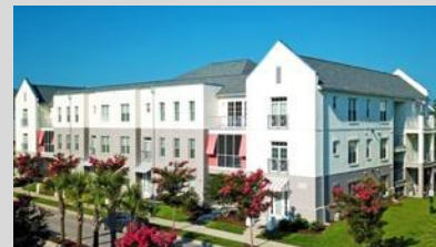
Link Apartments SM Mixson Charleston, SC 358 units
