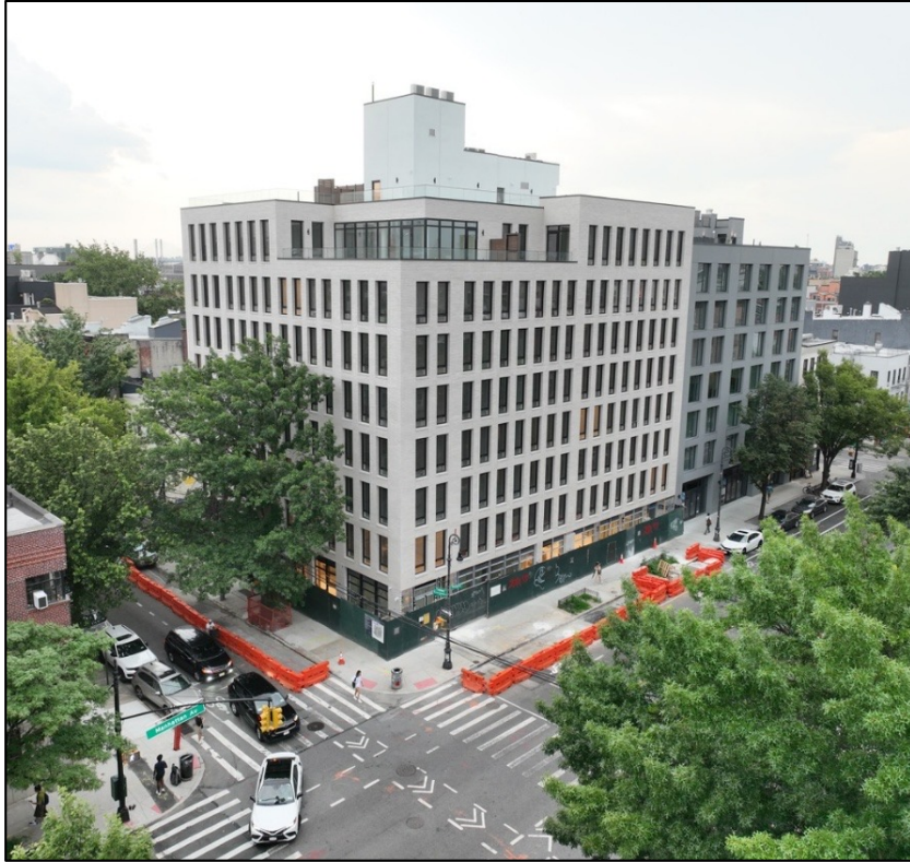
170 Freeman Street, Greenpoint (68 units)
