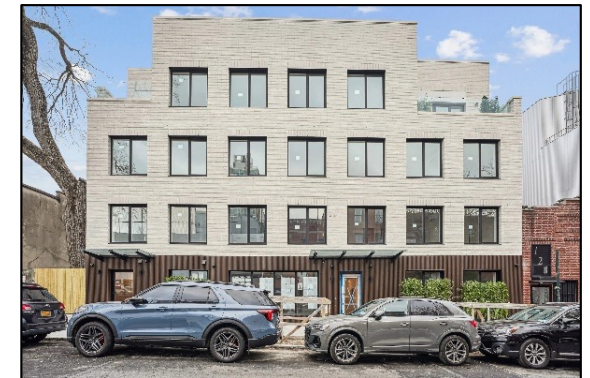
132-134 Waverly Avenue Clinton Hill (15 units)
